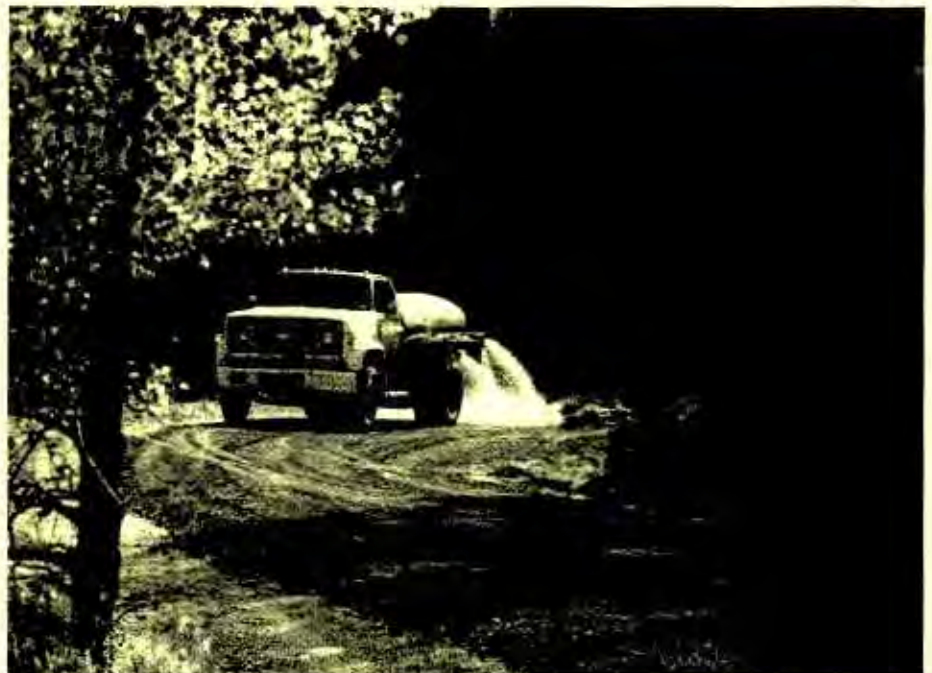
The RLA's new 1400-gallon tanker truck spraying water on freshly applied recycled asphalt on Miller Fork Road, September 19, 2000. More photos on page 3.
