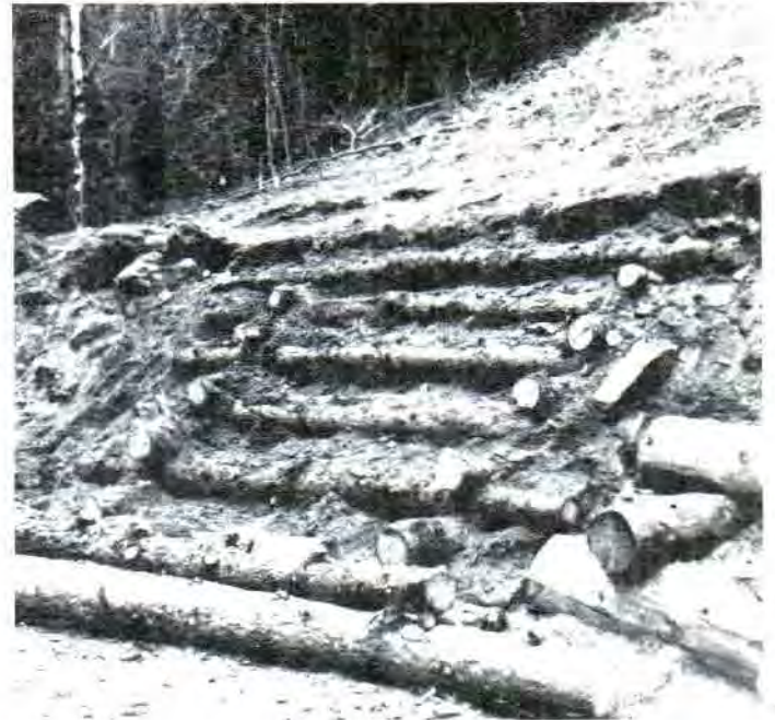
ATTRACTIVE AND EFFECTIVE erosion control measures are featured here. At left, rip-rapping around culvert faces and driveway banks prevents run-off and cutting (Mr. and Mrs. John Carroll, 12, F. 2). Above right, Mr. and Mrs. Ken Pitman are in the process of terracing an embankment on their property (10, F. 2) to preserve rich top soil.
