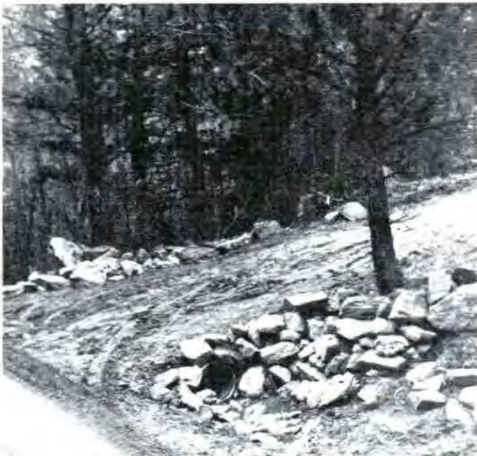
ATTRACTIVE AND EFFECTIVE erosion control measures are featured here. At left, rip-rapping around culvert faces and driveway banks prevents run-off and cutting (Mr. and Mrs. John Carroll, 12, F. 2). Above right, Mr. and Mrs. Ken Pitman are in the process of terracing an embankment on their property (10, F. 2) to preserve rich top soil.
