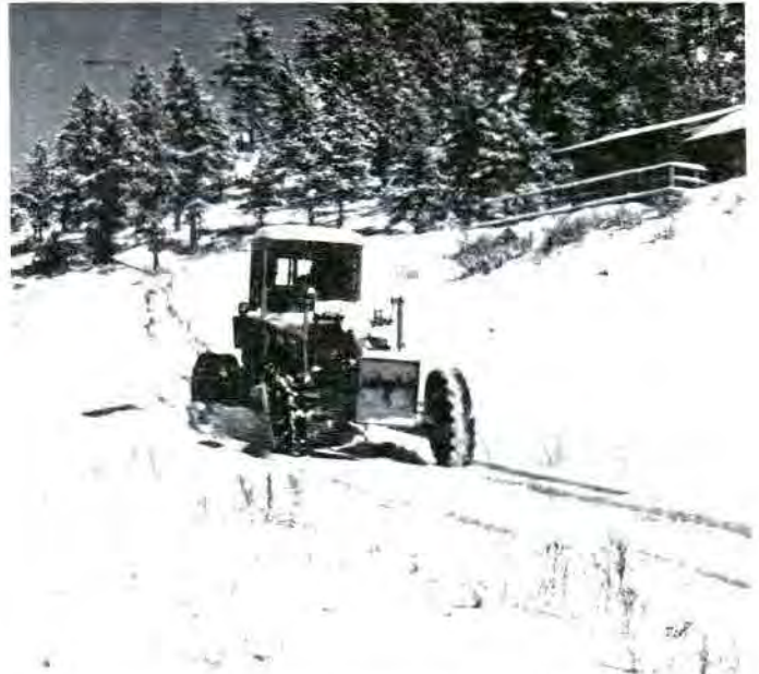
Retreat roads were plowed immediately after each new snowfall. Regular plowings prevent any ice layer from forming as a result of back-to-back snowfalls.
